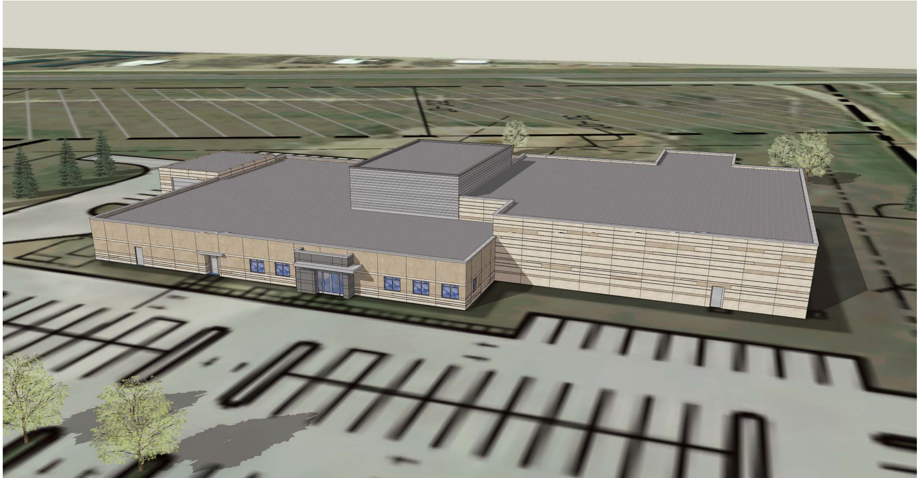
View of Public Entry from Stony Road (Facing West)
