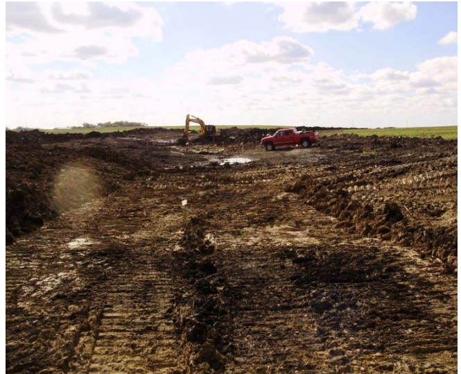
Shaping the bottom of waterway and side slopes. Average top width was 80ft. bottom width 20ft. with 8:1 side slopes.
