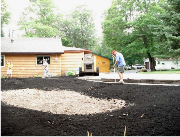
Final grading and landscaping before plants are placed.
