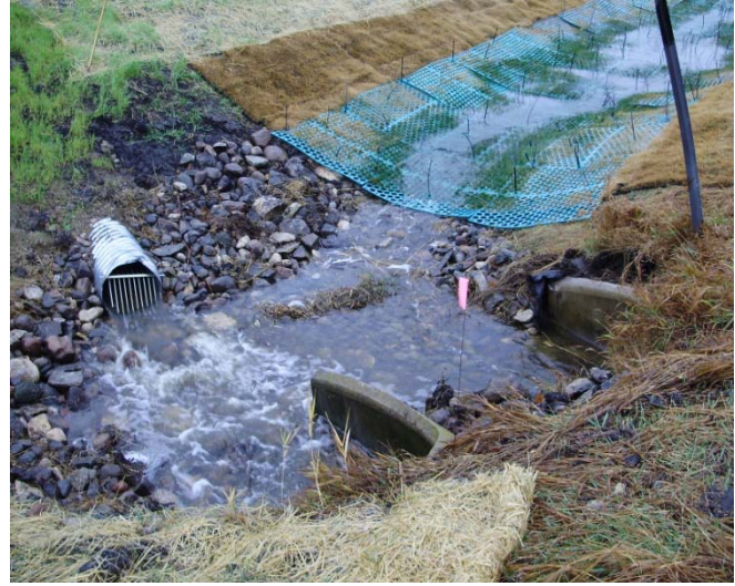
Completed outlet under Hwy. 59.
