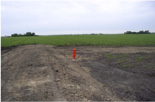
Typical tile inlet and dike of a water and sediment control basin.
